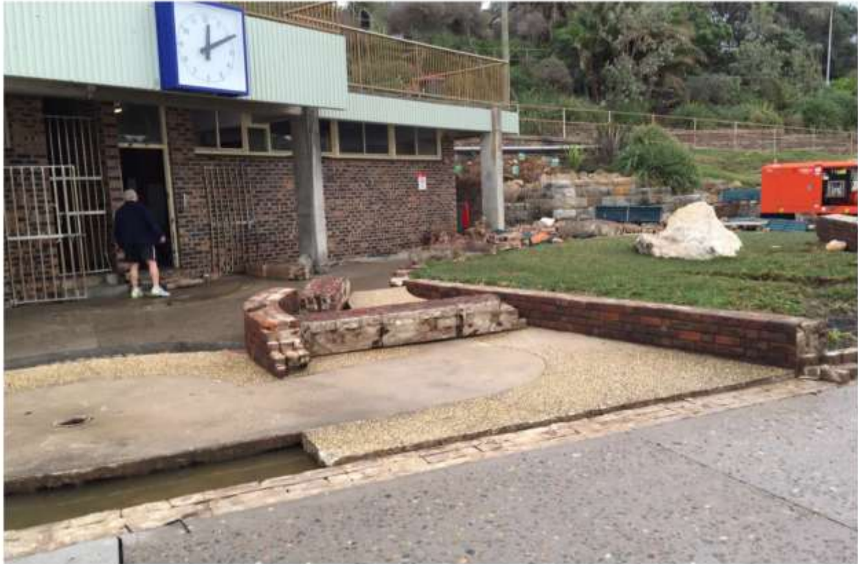
Figure 2 shows some of the damage to the retaining walls and metal doors at South Bronte Amenities (Horton Engineering)
