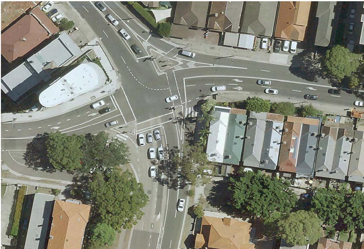
Figure 1. Intersection of Bondi Road and Council Street, Bondi Junction.
