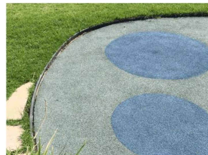
Photo 3: Existing worn rubber soft fall - slumping & separating from edging
