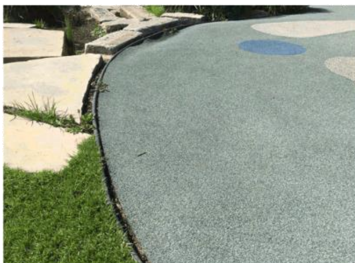
Photo 1: Existing worn rubber soft fall - slumping & separating from edging
