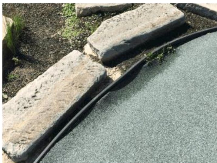
Photo 2: Existing worn rubber soft fall - slumping & separating from edging
