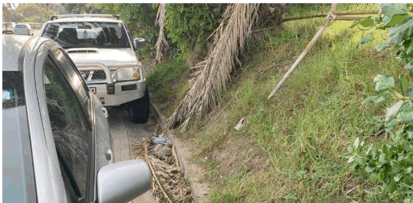
Image: Steep verge areas on Military Road will require localised earthworks and low walling to enable pedestrian path construction. To specific areas removal of parking is required to continue path
