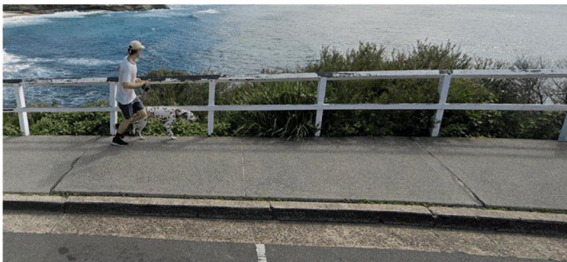
Figure 3-2: Existing footpath settlement and separation from kerb
