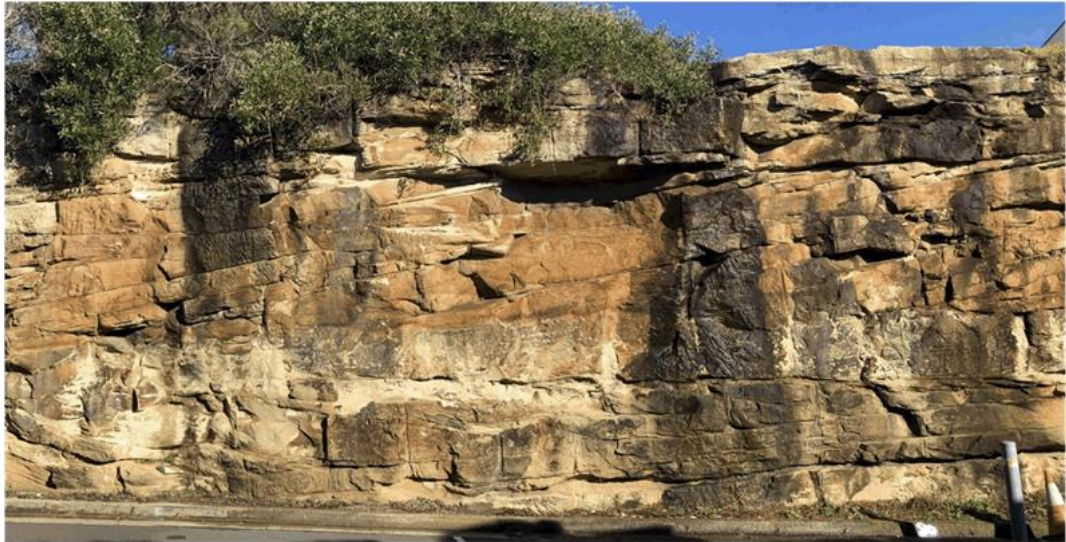
Figure 2-10 - Typical cutting face and small overhang
