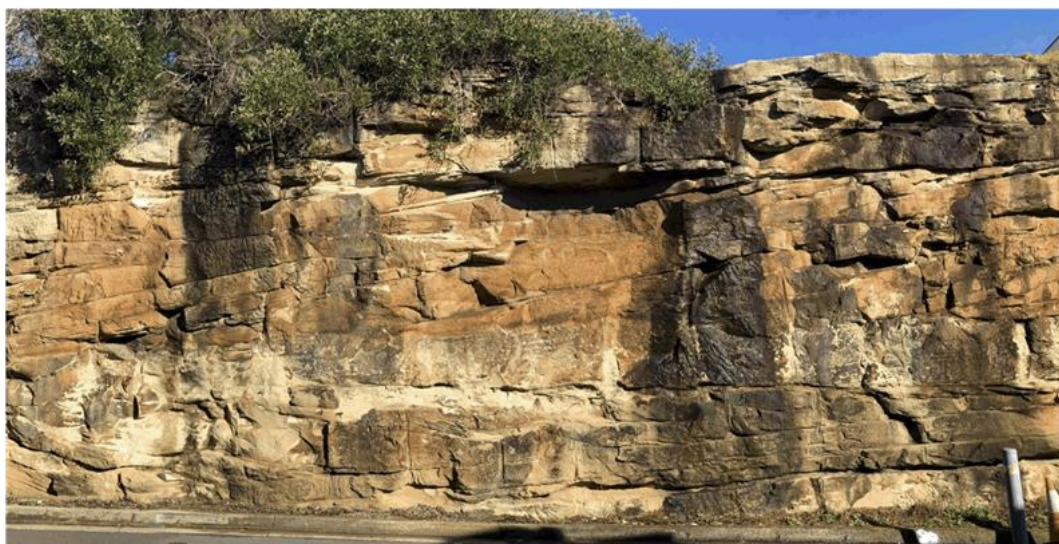
Figure 2-10 - Typical cutting face and small overhang
