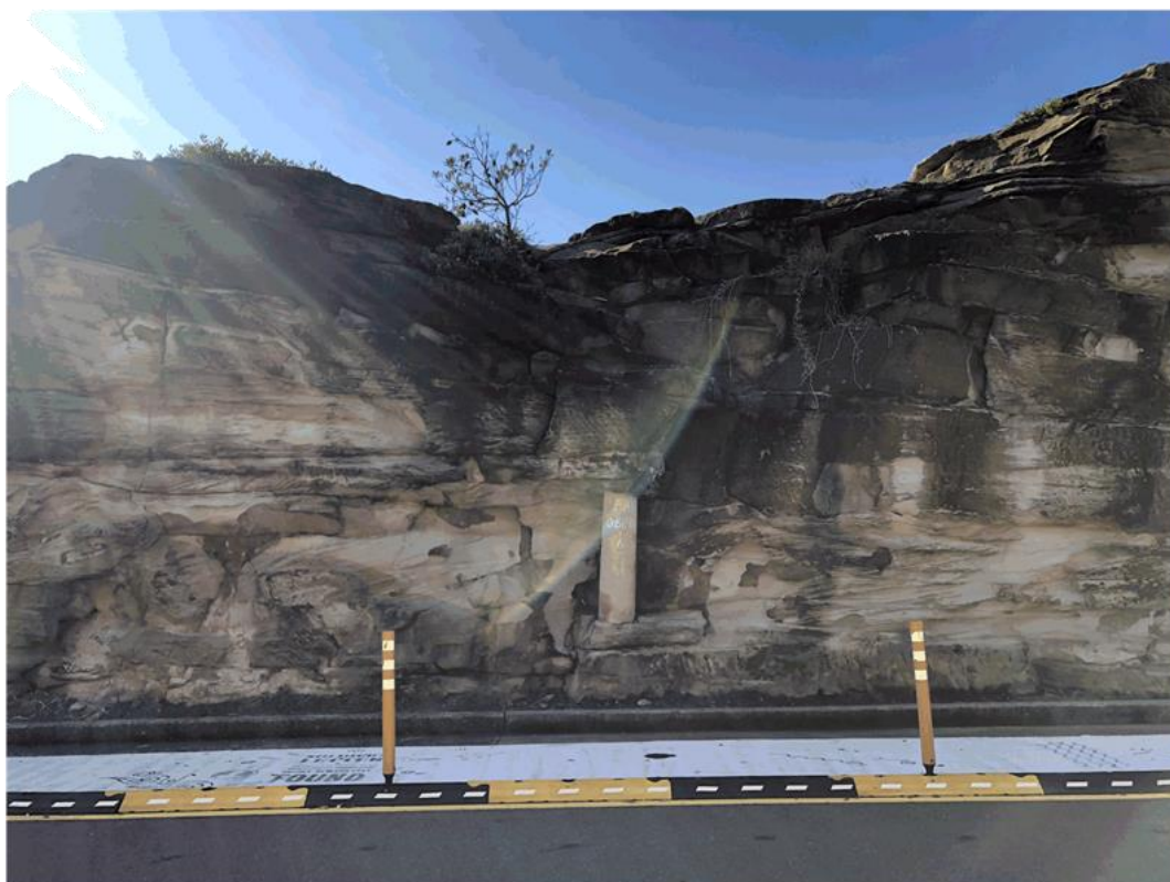
Figure 2-11 - Preferentially weathered beds and underpinned overhang
