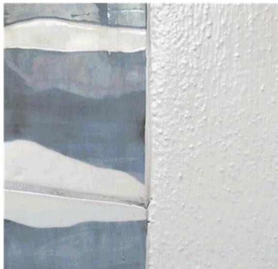
Figure 6. Tiles set into and flush with wall surface
