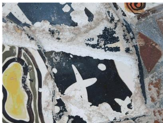
Figure 8. Highlighting loss of glaze
