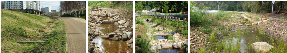
1 Infiltration swale with checkdams
