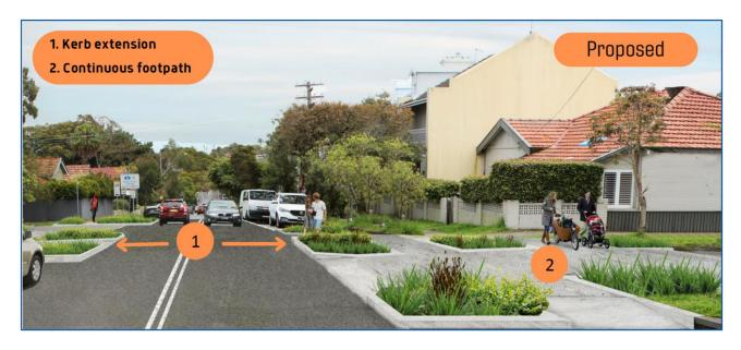
Figure 4. Birrell Street at Stanley Street – Replace pedestrian refuge with kerb extensions.
