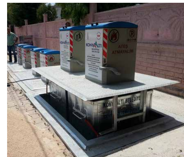
Hydraulic underground bins.
