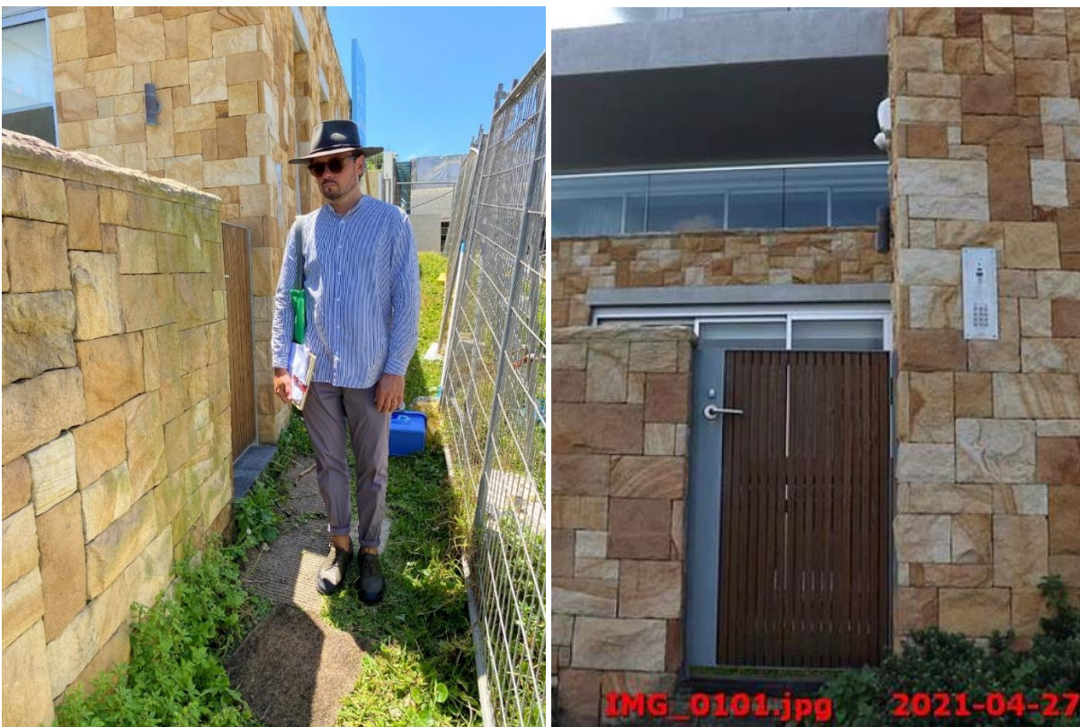
Figure 4. The boundary fence at 21 Gaerloch Avenue measures 1,510 mm adjacent the fitness equipment below the permissible 1,800 mm height. Buffer planting along the boundary has been trampled by visitors access the ground floor apartment.
