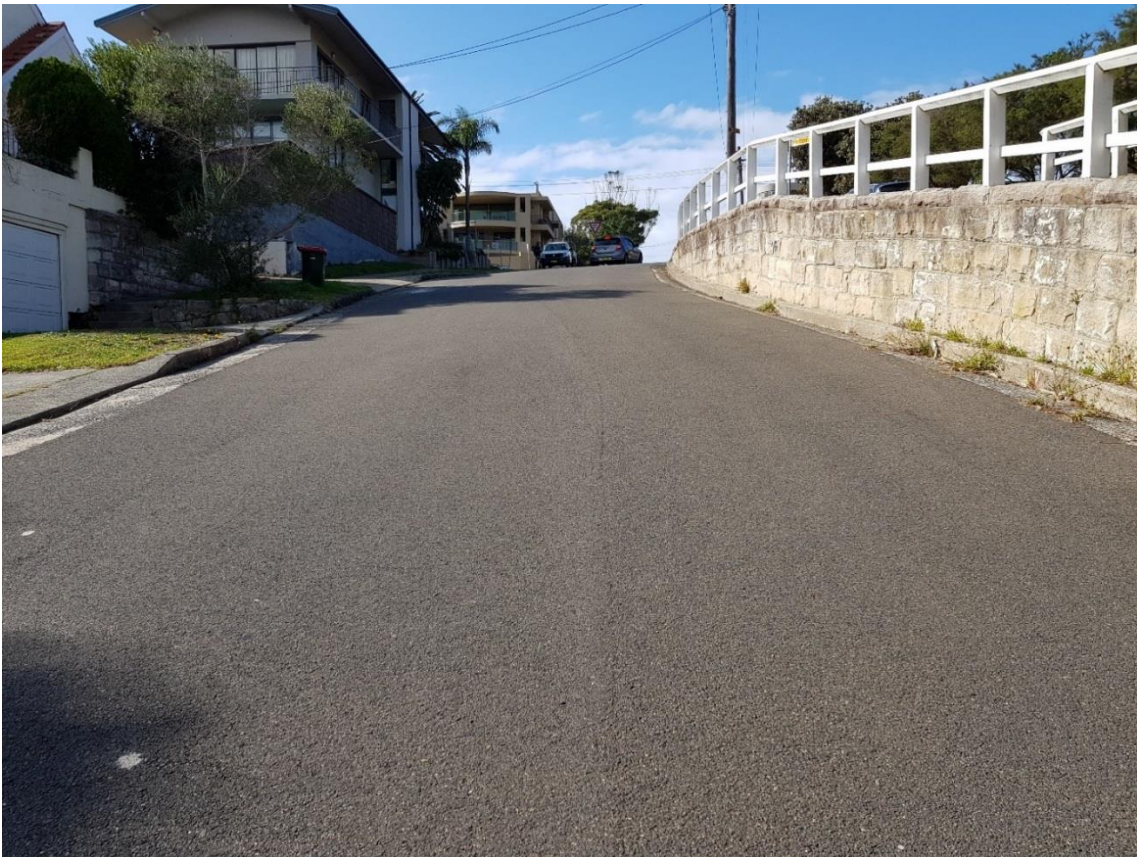
Figure 10. View of the intersection approach from Blake Street travelling east and the retaining wall obstructing the view of Victory Street.
