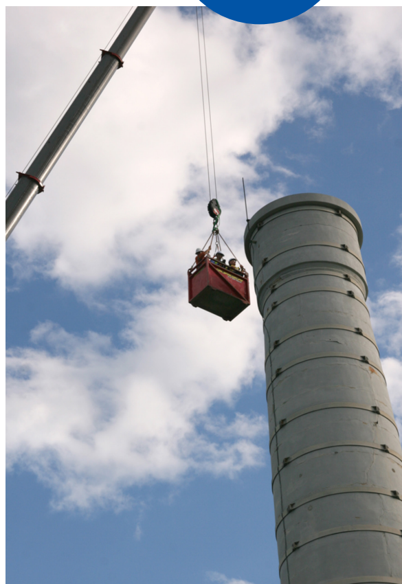
Our crews doing an external condition assessment of the Ben Buckler Shaft.
