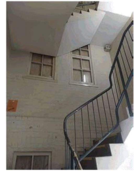
Concrete fire stair constructed in 1984.
