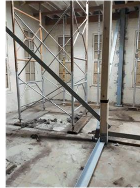
The interior of the building is currently compromised by remedial structural bracing members.
