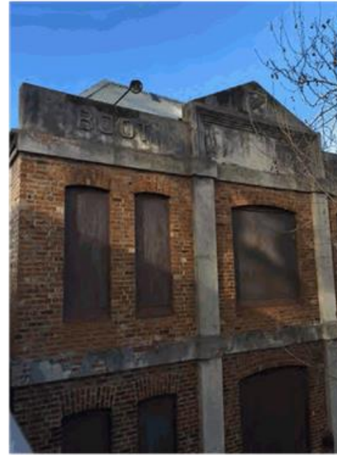
The windows are currently boarded up. Some exterior damage to render is visible.
