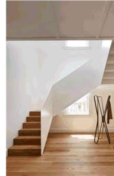
Staircase: Plate steel balustrade
