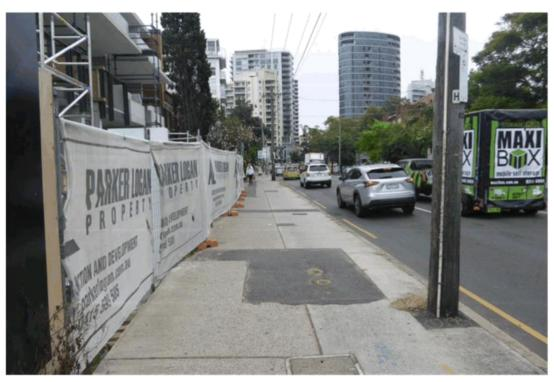
Photo 2: Damage to path surface adjacent to 91-93 Old South Head Road.
