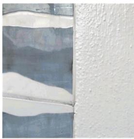
Figure 6. Tiles set into and flush with wall surface
