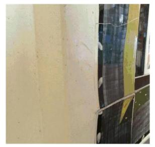
Figure 5. Tiles set into and flush with wall surface
