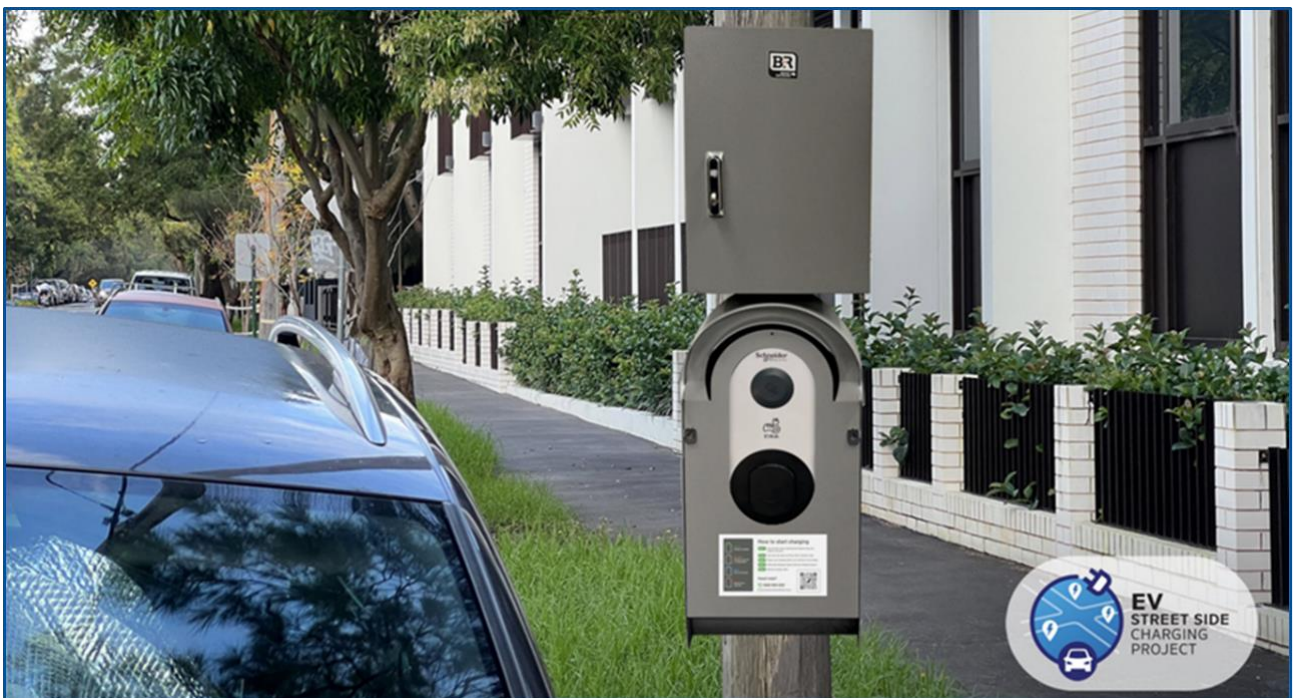
Figure 2. Street pole electric vehicle charging station (source: Intellihub).
