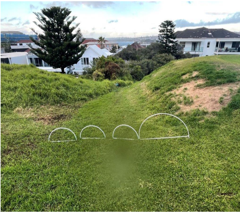
Figure 1. Opening between the two man-made hills which allows stormwater to exit into the rear garden of 146.
