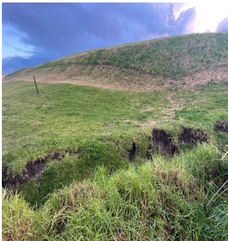
Figure 3. Gaping hole created by the stormwater.
