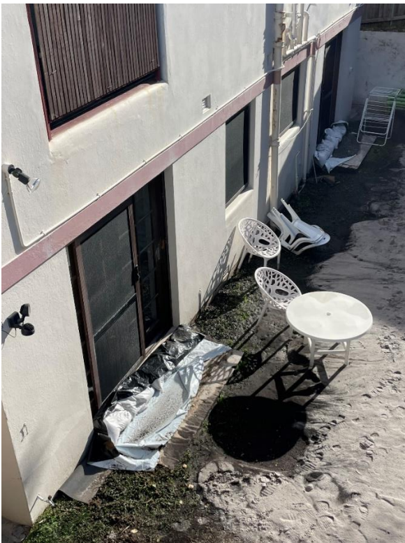
Figure 9. Apartments at ground level have sandbags to permanently protect rear doors.
