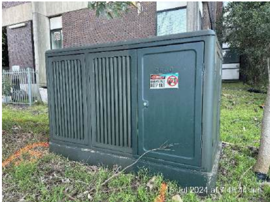
Electrical Padmount Station located on subject property
