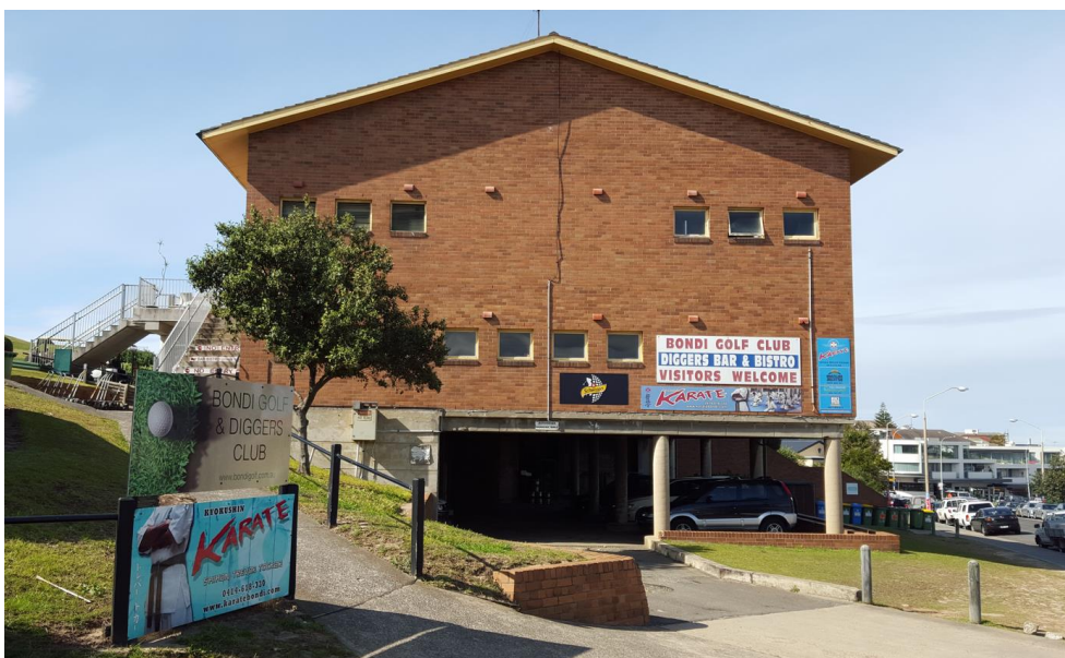
Figure 2. Bondi Golf and Diggers clubhouse building.
