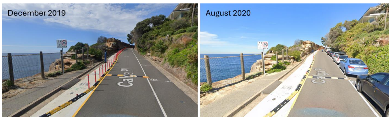
Figure 2. Calga Place temporary collapsible delineators with considerable wear and tear.
