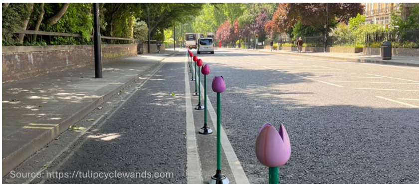
Figure 4. Tulip cycle wands installed in the UK.
