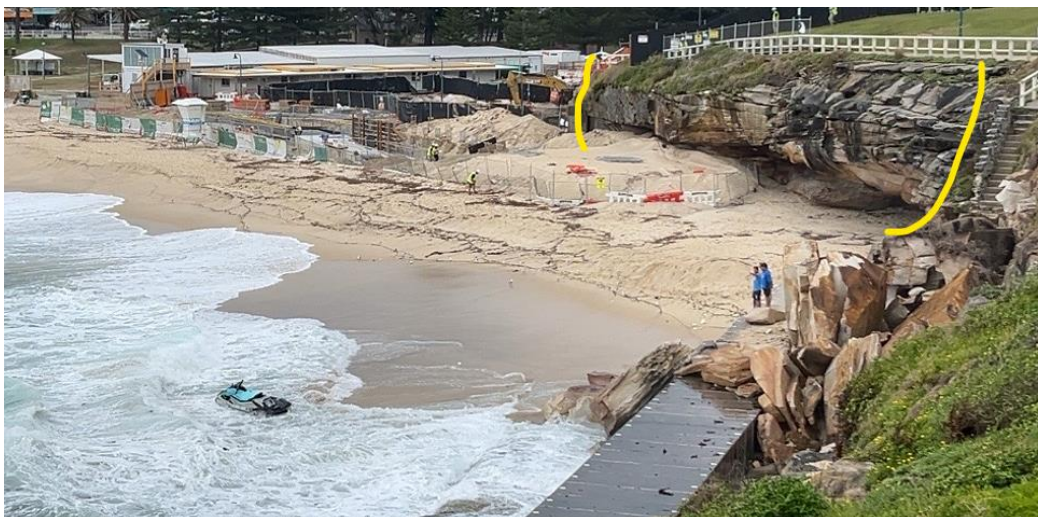
Figure 3. North Bronte Park – Cliff inspection – Area B.
