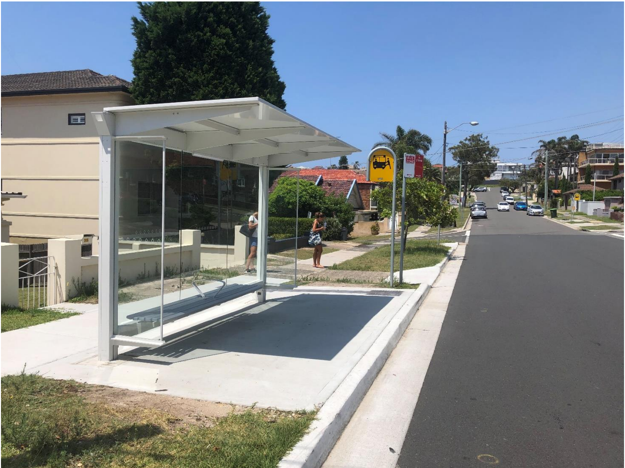
Figure 1. Bus stop at 305 Military Road.
