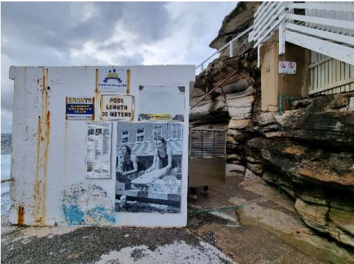
Figure S22 – Association of the pumphouse and cliff-face. Note the large concrete ‘pillar’ on the cliff-face supporting the cliff stair.
