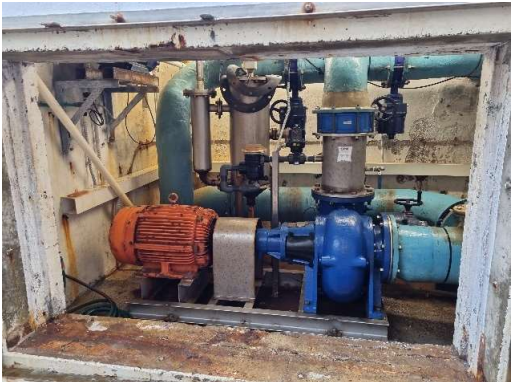
Figure S26 – Pump machinery viewed through the access doors on the south-western elevation of the pumphouse.
