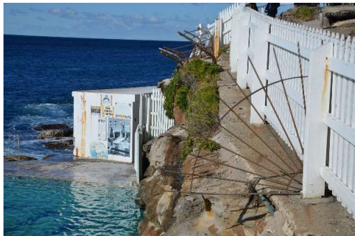
Figure S9 – The western façade of the pumphouse building facing the ocean pool. Note the various public safety accretions of occupance on the cliff face, including barbed wire, to discourage public access and jumping into the pool.
