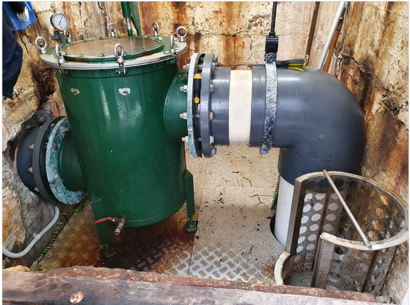
IMAGE 2 - PLATFORM AND BASKET STRAINER ABOVE PUMP SUMP
