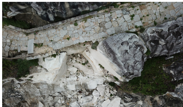
Repairs on the coastal walk beneath Marks Park
