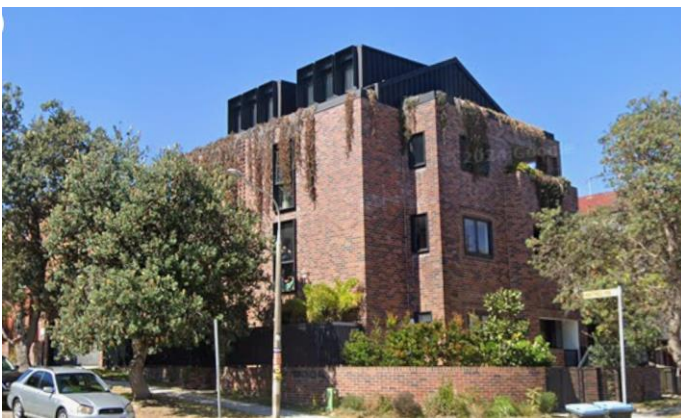
Figure 1. Inter-War building at 1 Hastings Parade, Bondi Beach with contemporary alterations and additions (source: Google Maps 2024).
